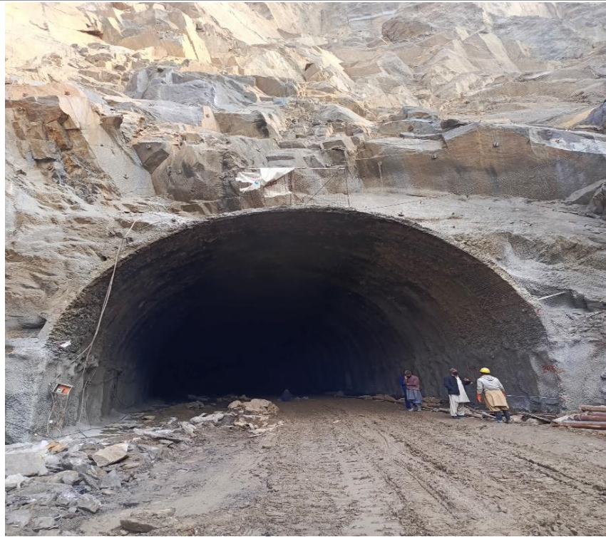
Figure 3: Excavated portal face of the Karakar Tunnel, showing the jointed, foliated schistose rock mass exposed prior to lining (site photograph, 2026).
